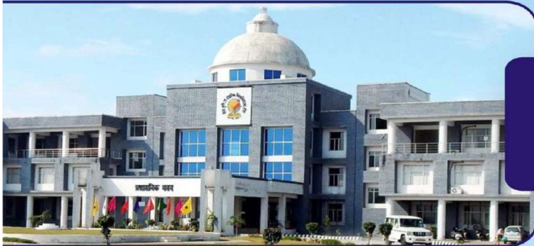
Administrative Building BUA&T, Banda
